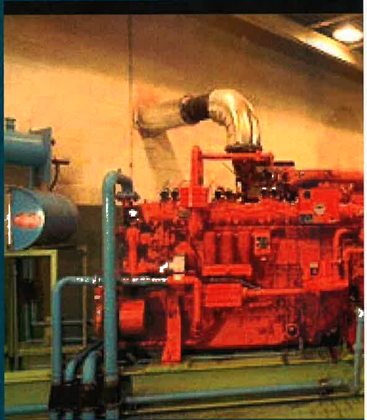
Waukesha VGF F18G drives 90 kW induction generator in parallel with utility for Canonsburg, Pennsylvania, wastewater treatment plant. Recovered heat is used to maintain temperature in digesters.
