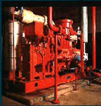
Waukesha VGF F18G drives 90 kW induction generator in parallel with utility for Canonsburg, Pennsylvania, wastewater treatment plant. Recovered heat is used to maintain temperature in digesters.
