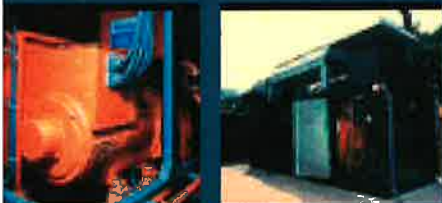
A landfill at Vlagheide in Schijndel, The Netherlands, has five H24GLDs efficiently generating electricity from low BTU landfill gas.
