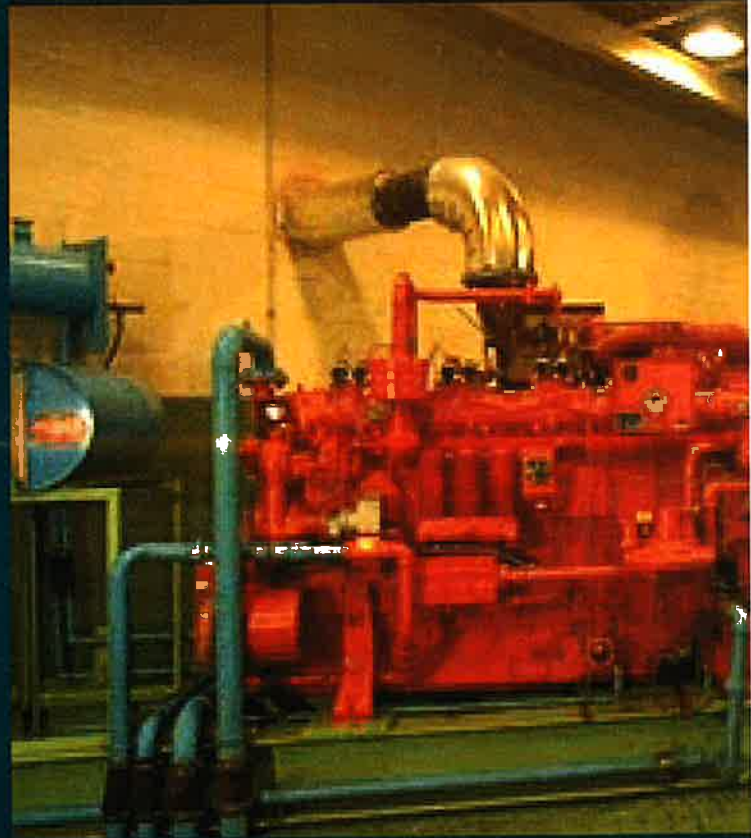
Waukesha VGF F18C drives 90 kW induction generator in parallel with utility for Canonsburg, Pennsylvania, wastewater treatment plant.
