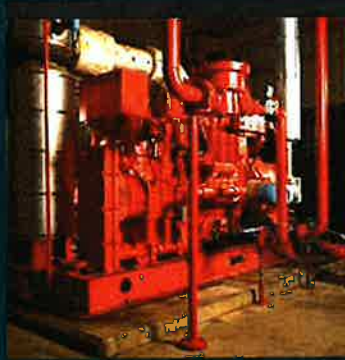
Waukesha VGF F18C drives 90 kW induction generator in parallel with utility for Canonsburg, Pennsylvania, wastewater treatment plant.
