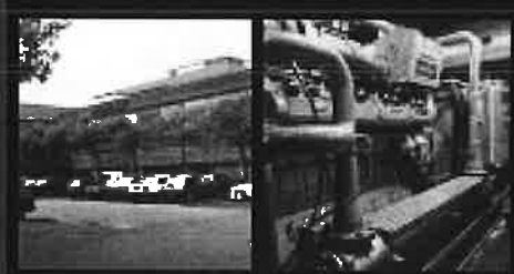
Elkerliek Hospital in The Netherlands uses a P48GLD and an H24GLD for standby power and cogeneration.
