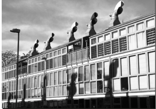
Photo of housing unit at BedZED with colorful wind cowls that help provide energy to the community. BedZED was featured in the award-winning film by the Ventura County Air Pollution Control District, Air – the search for one clean breath .
