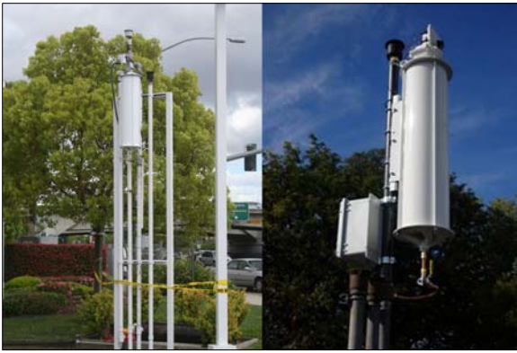
Carbon canister-type EVR system
