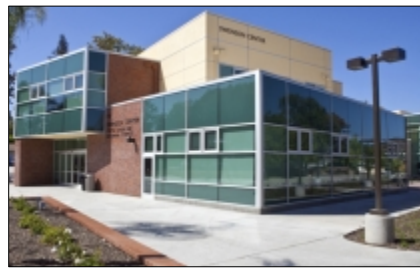
CLU's new $8.5 million LEED certified "green" building, the Swenson Center for the Social and Behavioral Sciences.
