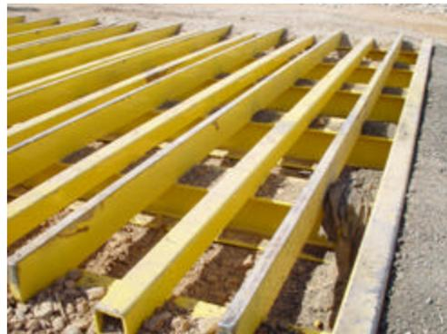
**Figure 5: Grizzly rumble grate used to prevent track-out.**
